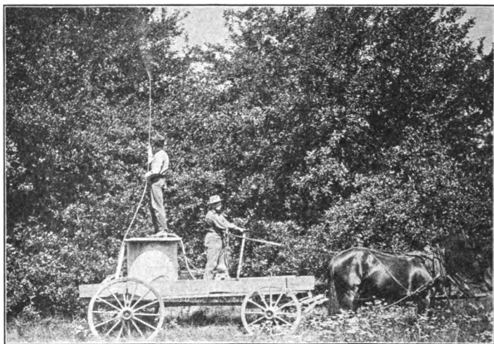
FIG. 307. — Suitable Spraying Outfit for a Small Orchard.
